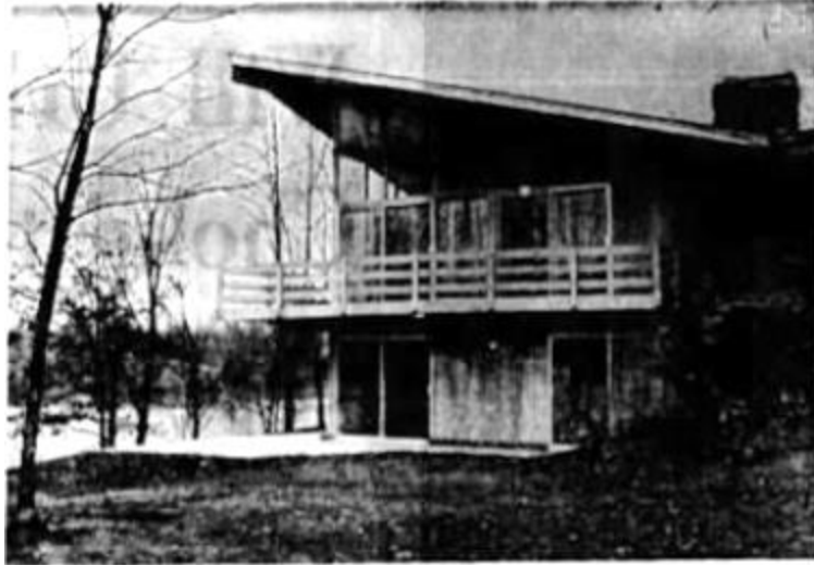
Roof of the home of Mr. and Mrs. A. B. Osswald on Crystal Lake at LaGrange, Ky., soars up and out above windows and gables of glass rising to a height of 15 feet. A balcony surrounds the living and dining areas. The house is built on an eye-catching three-acre lot.
