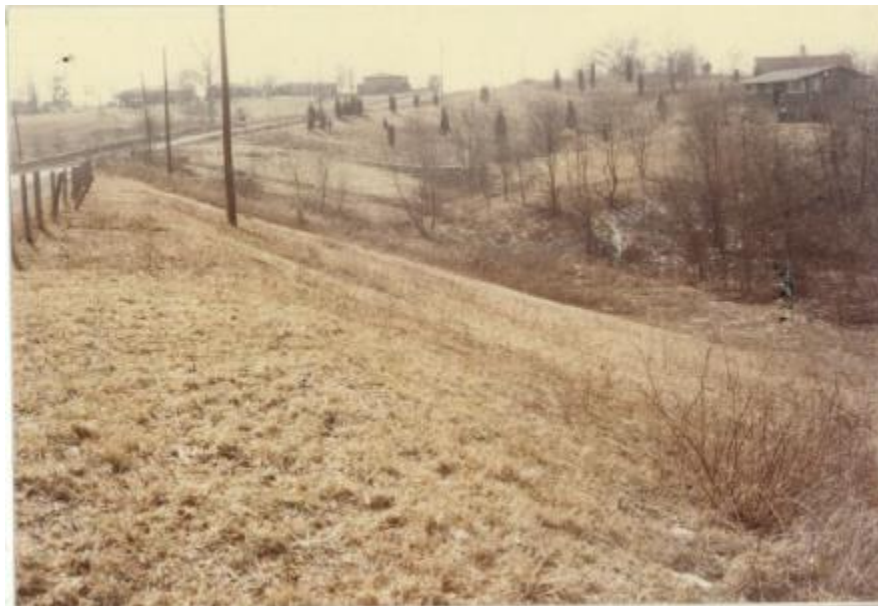
Figure 11 Crystal Lake Dam Toe
